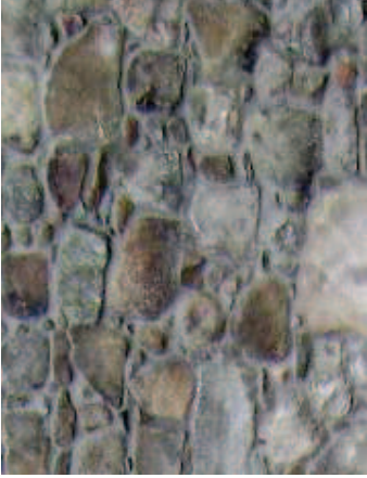
G Granite rubble masonry.
